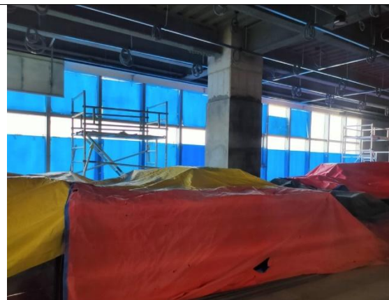
Figure 2.8 Storage room for construction material
