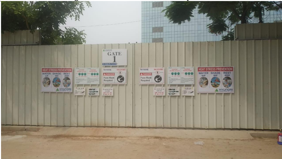
Figure 2.10. Barricading and safety boards
