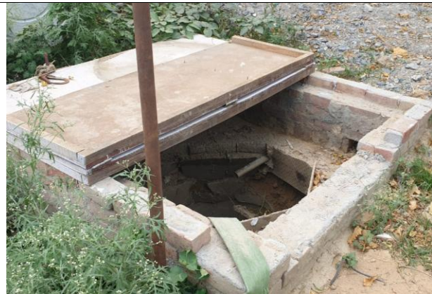
Figure 2.6 Rainwater Harvesting pit under construction
