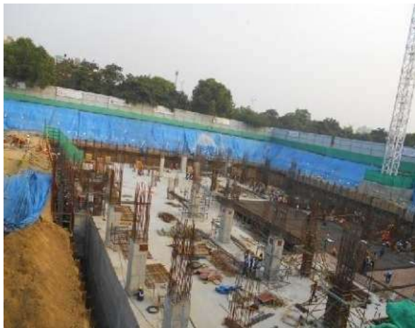
Figure 2.1. Showing construction status
